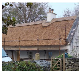
THATCH WORKS COMPLETED AT TURLOUGHMORE AND LOUGHCURRA SOUTH
