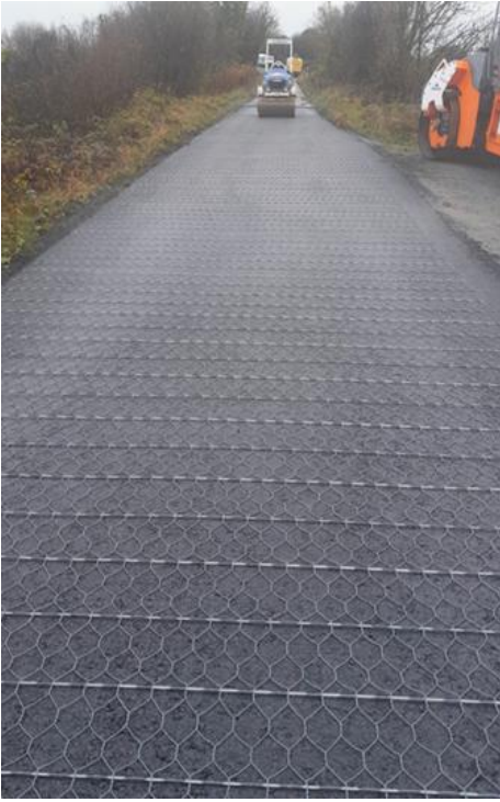
ROAD REMEDIATION WORKS FOLLOWING PREMATURE LOCALISED ROAD FAILURE AT KILLORAN, LOUGHREA
