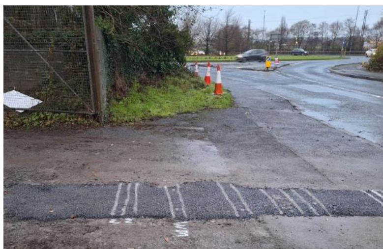
SLIT TRENCHES – STATION ROAD ORANMORE
