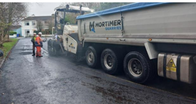
WORKS AT CONVENT PARK HOUSING ESTATE, KINVARRA
