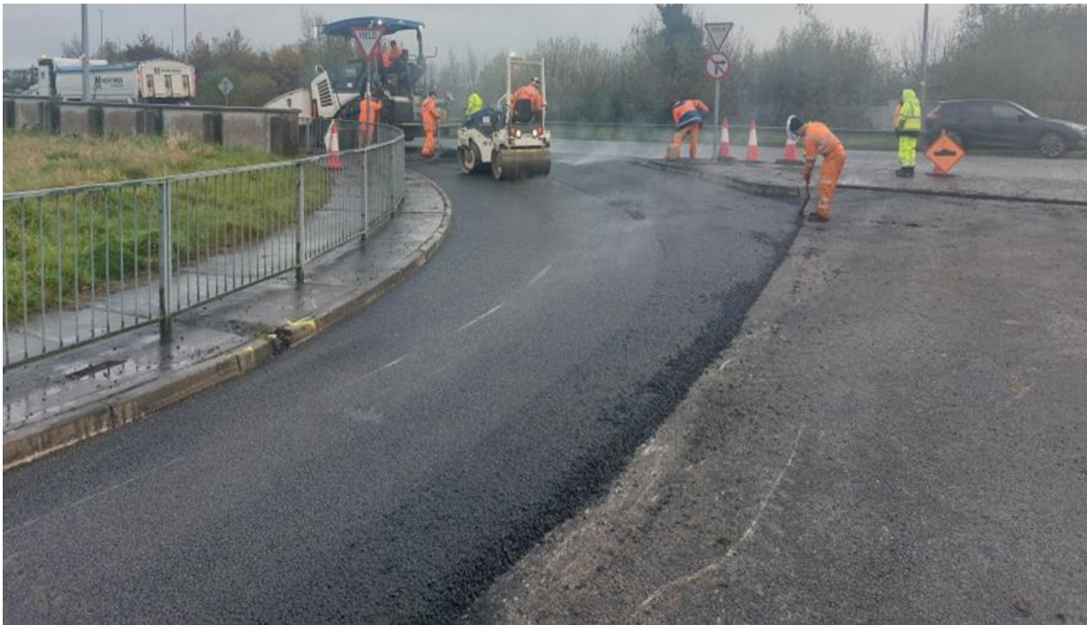
ROAD RESURFACING WORKS AT COSMONA, LOUGHREA
