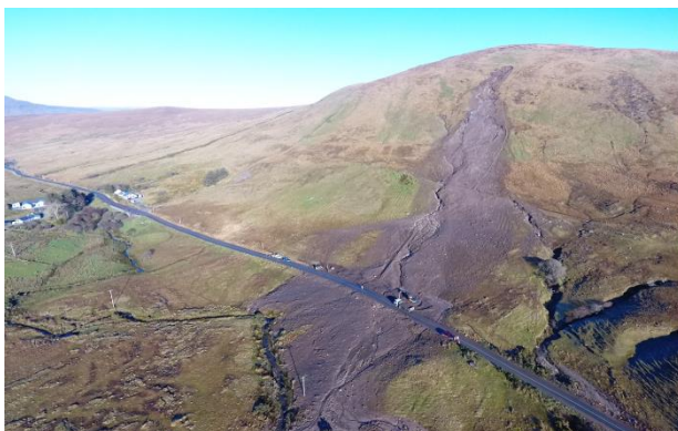
R336 MUINTIR EOGHAN STORM BERT LANDSLIDE DURING CLEAN UP
