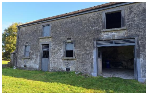
MASONRY REPAIR WORKS COMPLETED AT CREGACLARE DEMENSE
