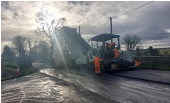
JUNCTION IMPROVEMENT WORKS ON THE N65 AT GURTYMADDEN
