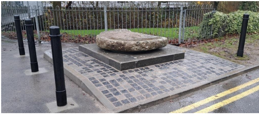
REPAIRS COMPLETED TO THE TYRING PLATFORM AT SAINT MICHAELS SQUARE, BALLINASLOE
